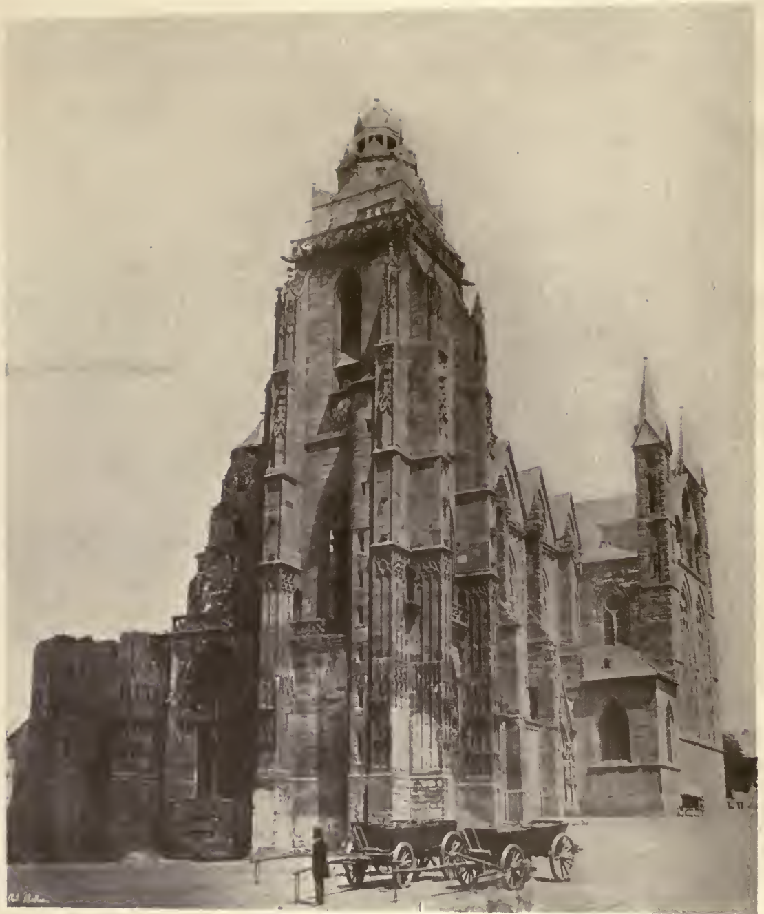
THE CATHEDRAL, WETZLAR, GERMANY
